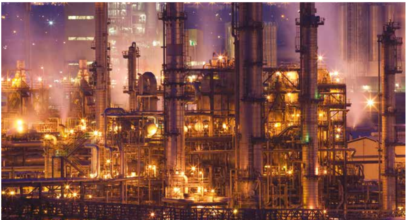
Grangemouth Oil Refinery
